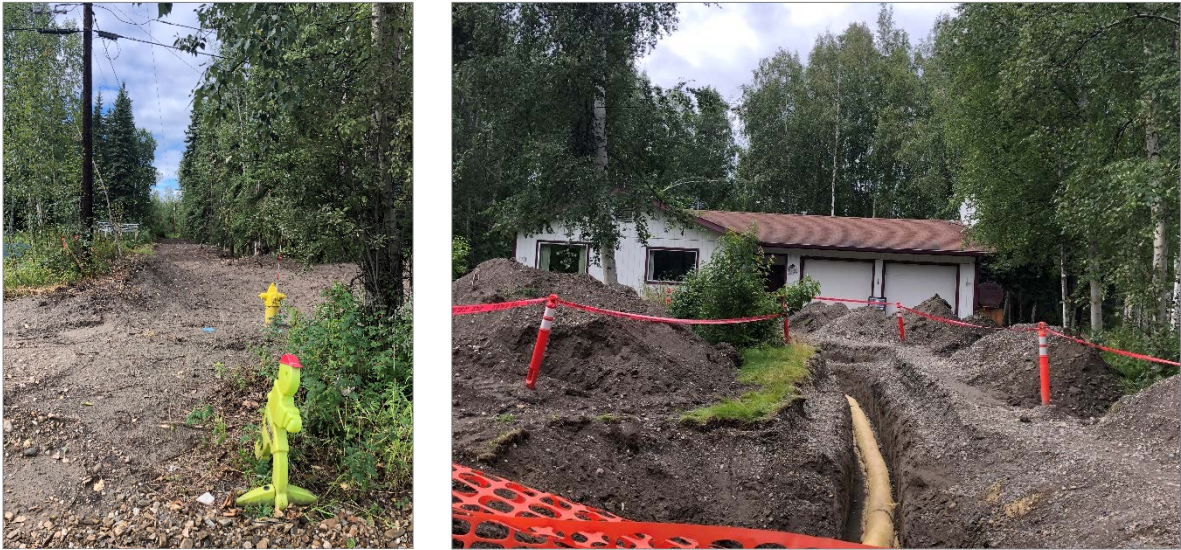
Exhibit 2-6: Photographs of Land Clearing and Newly Installed Water Line
